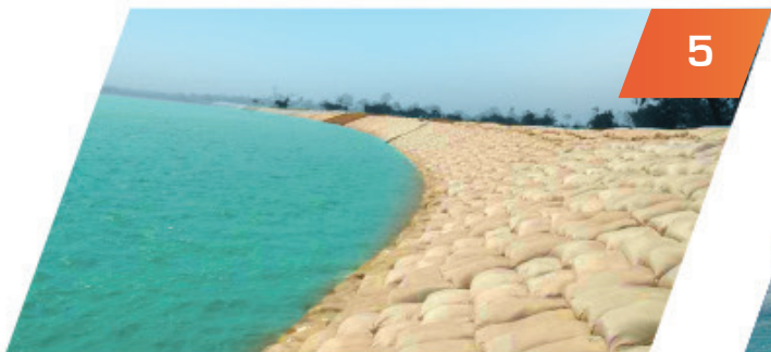
SAND TUBE & SAND BAGS PROTECTION WORKS
